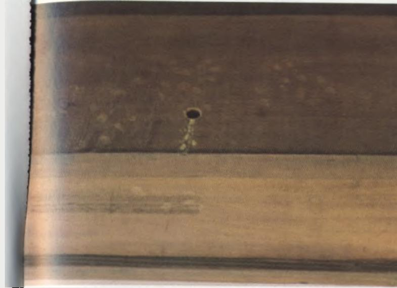
Figure 50. Carpenter bee entry hole (approximate diameter 1/2 inch) with streak of fecal matter below
