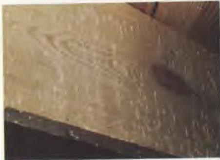
Figure 39. Anobiid damage with powder streaming from insect exit holes
