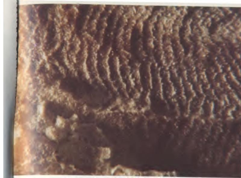
Figure 47. Typical etching wall of old house borer gallery
