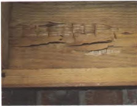
Figure 11. Wood damaged by *Poria*, with apparently sound surface and severe rot below surface
