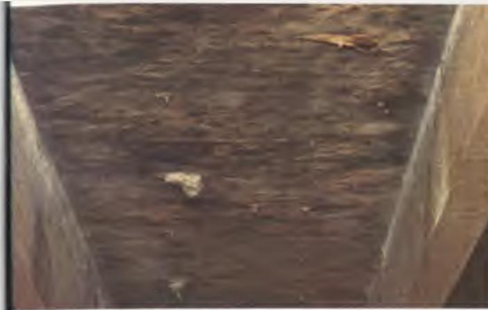
Figure 4. Surface molds on plywood in attic
