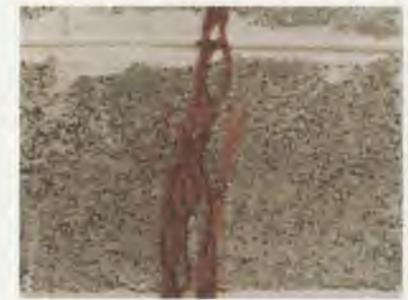
Figure 19. Subterranean termite shelter tubes on concrete block foundation wall
